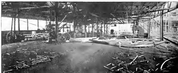
The bending slabs, Harlan
